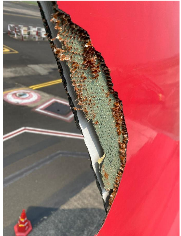
Close-up of damage to VT-TGG
