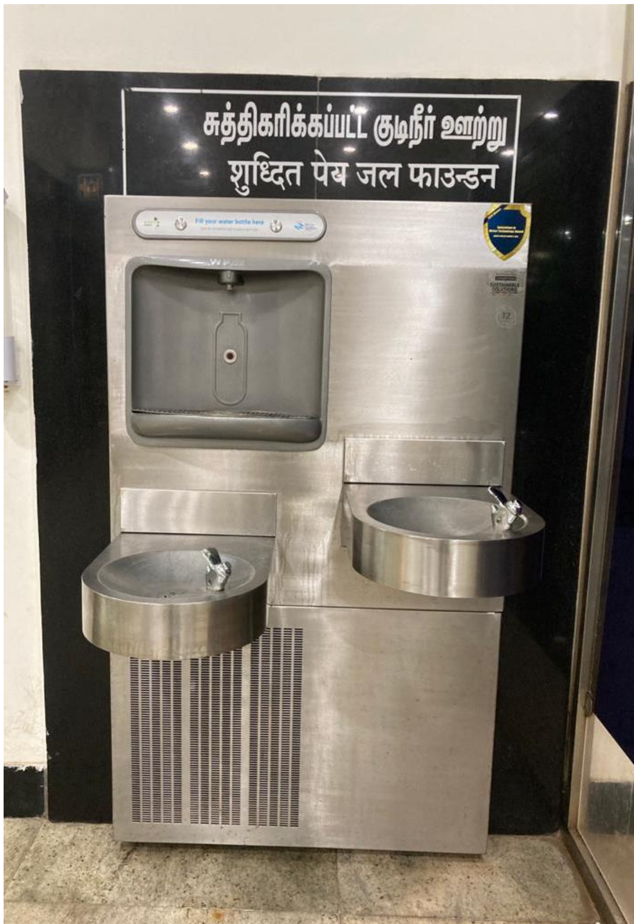
Image 16: Example of Drinking water facility with taps on two levels installed in Madurai Airport
