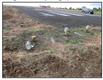
Fig. 07. Damage to RWY 27 end light
